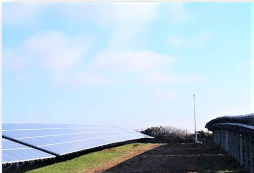
Image 5. Bare earth or poor grass regeneration on the working area within the shadow line.
