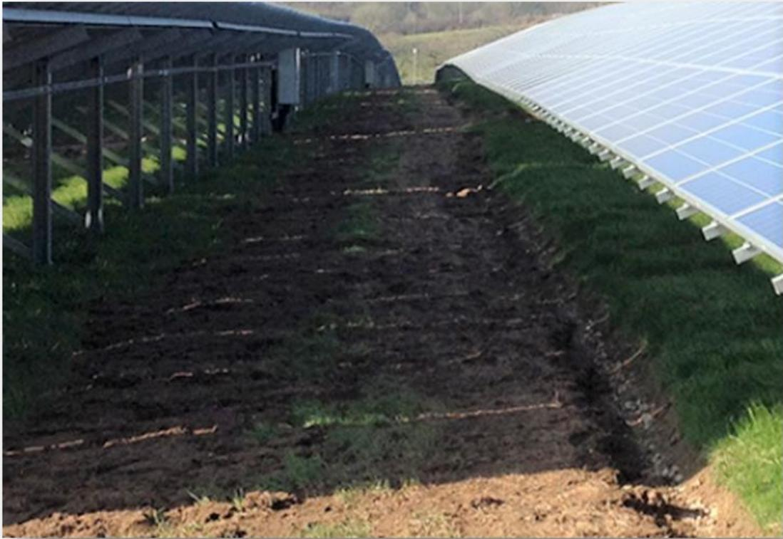
Image 4. Shows very poor grass cover on the worked-on area. Lower right clearly shows the ground scouring caused by rivulet run-off from the lower edges of the solar panels. The kinetic energy of the water draining from the solar panel could be as much as 10 times greater than that of rainfall. (Cook and McCuan 2013)
