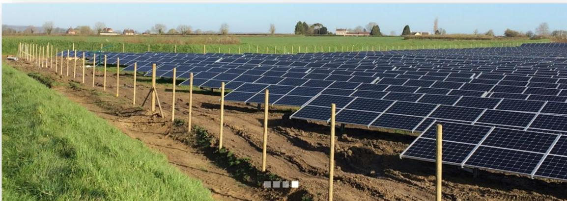
Image 7. BSR site Southfields. Repairing grass cover after construction damage and compaction might not take place until the following spring (as soil temperature would be too low for grass germination) leaving the site particularly vulnerable to flooding and increased runoff during that period.
