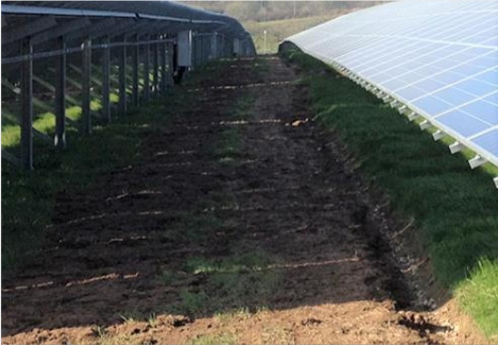
Image 1. Shows very poor grass cover on the worked-on area. Lower right clearly shows the ground scouring caused by water runoff from the lower edges of the solar panels. The kinetic energy of the water draining from the solar panel could be as much as 10 times greater than that of rainfall. (Cook and McCuen 2013)
